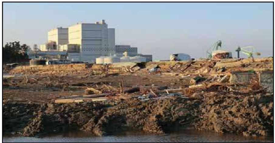
Figure 3: The damaged power plant at Fukushima
